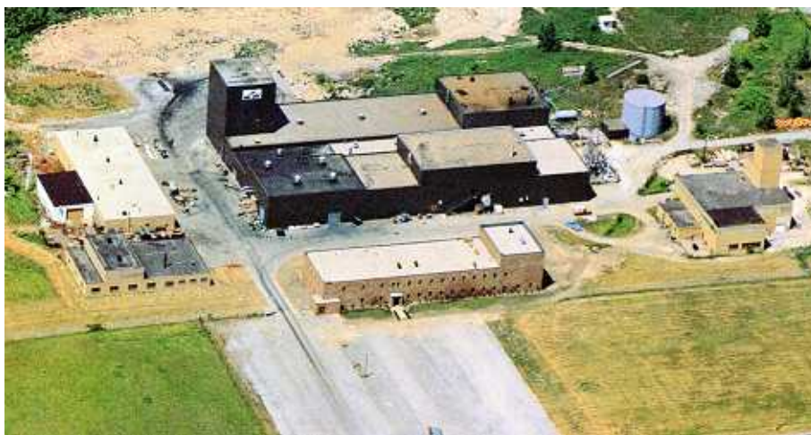
Engineering, manufacturing, administration & customer service are housed within I 2 R wholly-owned 90,000 softcomplex at Akron, NY, U.S.A.
